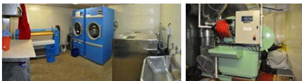
Laundry; Incinerator (Garbage burner).
