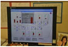
Tank control of fuel, lubrication oil, bilge-, fresh- and ballast-water.
